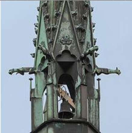
Copper belfry of St. Laurentius church, Bad Neuenahr-Ahrweiler
